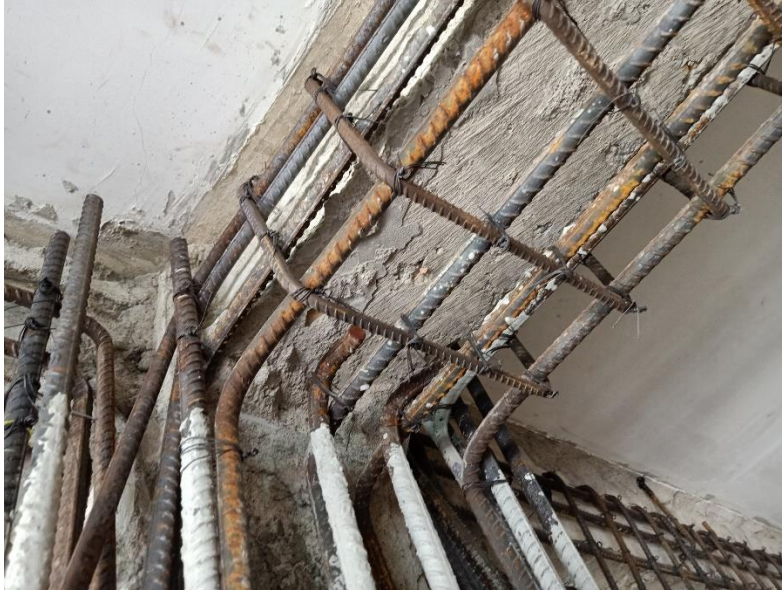
Gambar 2. Concrete Jacketing proyek Mamuju
